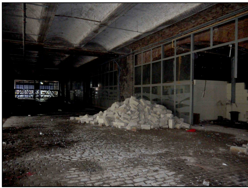
JACK ARCHES UP TO LONDON ROAD - This significantly contributes to the character of London Road and is generally to be retained.
